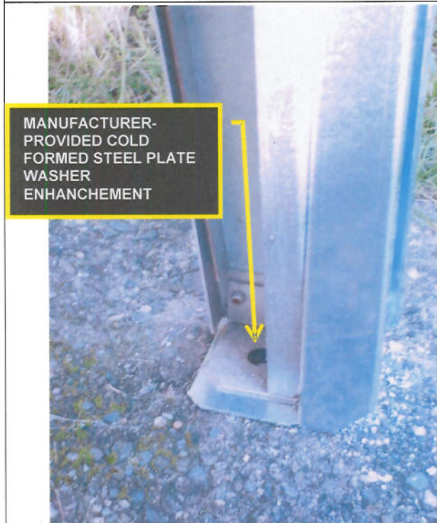
Photo 3: Anchor Point Reinforcing
