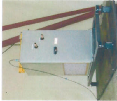
42DFA06, suspended with HRS-1C hanger boxes
