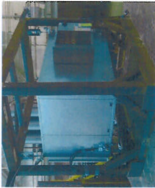
42CKA12, suspended with HRS-1C hanger boxes
