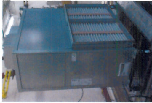
42BVD40, Base Mounted on AMSR-1C Isolators
