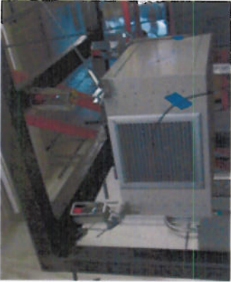
42DFA06, suspended with HRS-1C hanger boxes
