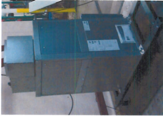
42BVD06, Base Mounted on AMSR-1C Isolators
