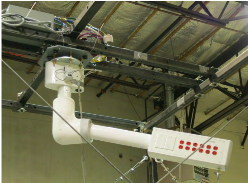
UUT2, mounted to test frame, instrumented and ready for test.
