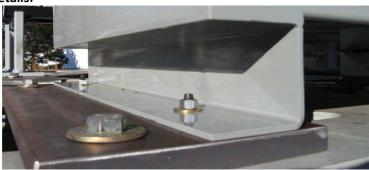
The unit was mounted to steel plates using four grade 8 3/8"-16 bolts with standard washers (two in each angle iron foot).
