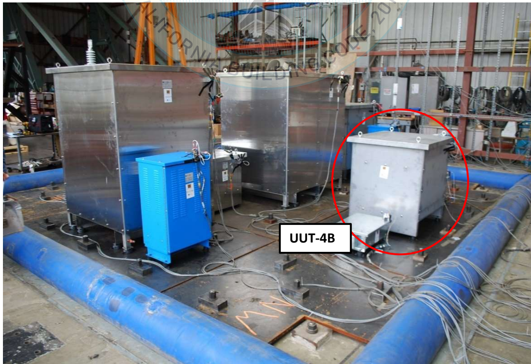
All units were filled with contents and maintained structural integrity and functionality after AC-156 test.
