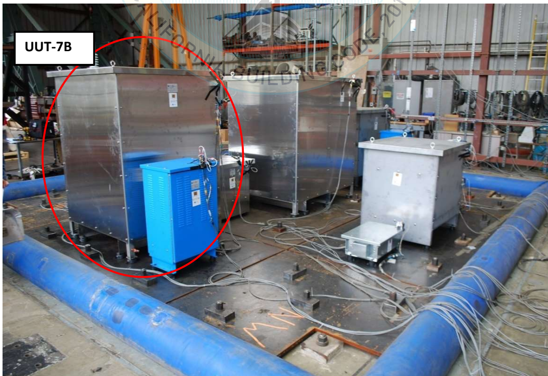
All units were filled with contents and maintained structural integrity and functionality after AC-156 test.
