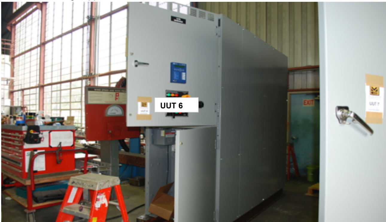
All units were filled with contents and maintained functionality and structural integrity
