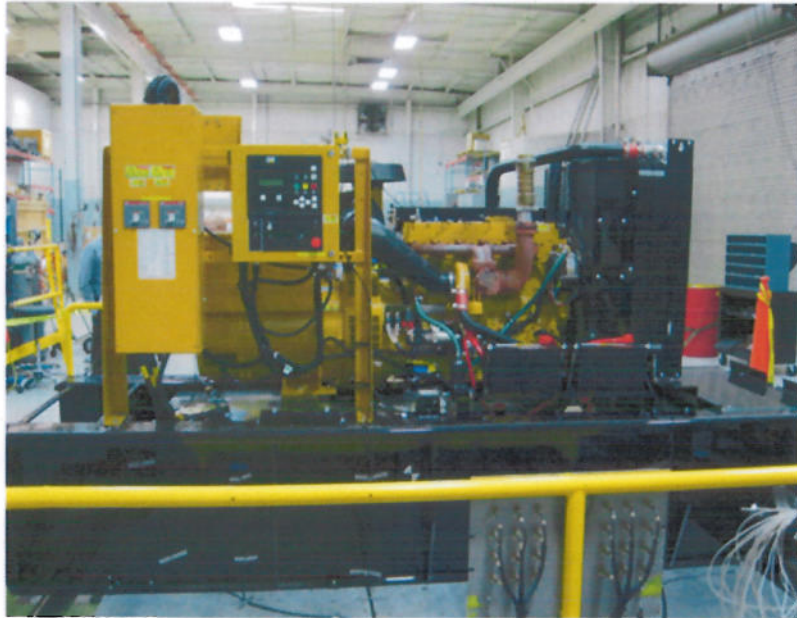
Tests #1 & #2, hard mounted on a tank
