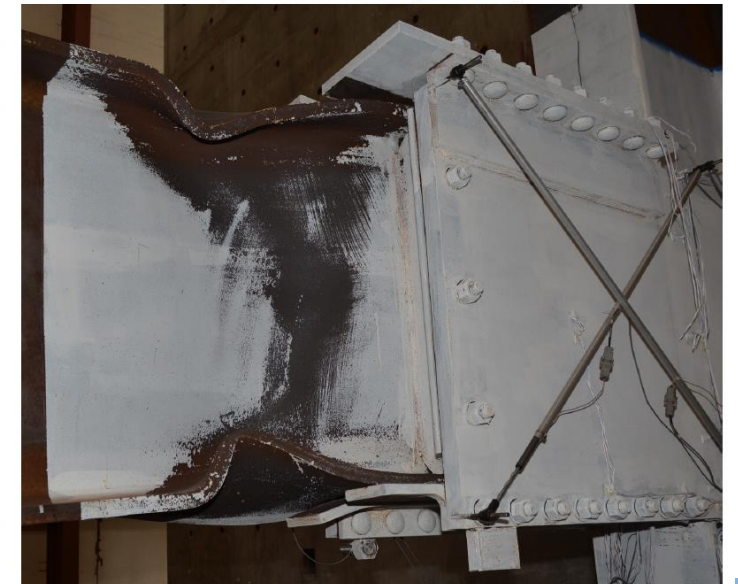
Beam Flange and Web Local Buckling (at Test Completion)
