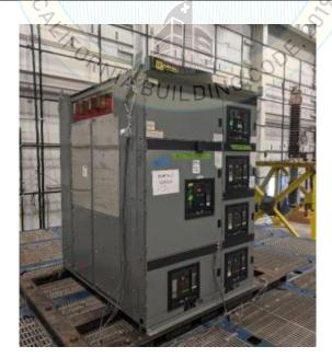
UUT was rigid base mounted using (8) 1/2"-13 Grade 5 bolts.
