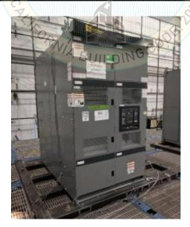
UUT was rigid base mounted using (6) 1/2"-13 Grade 5 bolts.
