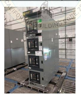
UUT was rigid base mounted using (4) 1/2"-13 Grade 5 bolts.
