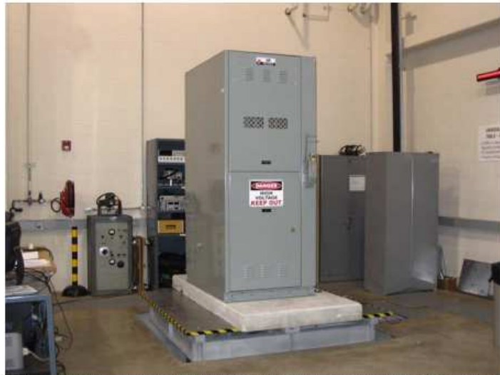
Figure 1-10: IEM Medium Voltage Switchgear Mounted to Earthquake Simulator for Vertical Vibration
