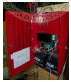
Unistrut was rigid mounted to a 5/8" fire-rated drywall covered wall fixture using (4) ungraded 3/16" toggle bolts. The unit was rigid wall mounted to unistrut using (4) ungraded 1/4" bolts into spring nuts.
