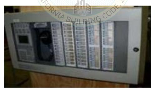
The unit was rigid wall mounted using two ungraded 3/16" toggle bolts through a 5/8" drywall covered wall fixture. Unit maintained structural integrity and remained functional per manufacturer requirement after shake table test. Contents were included in testing per operating conditions.
