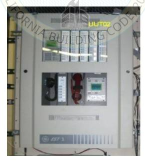
Unistrut was rigid mounted to a 5/8" fire-rated drywall covered wall fixture using (6) ungraded 3/16" toggle bolts. The unit was rigid wall mounted to unistrut using (4) ungraded 1/4" bolts into spring nuts.
