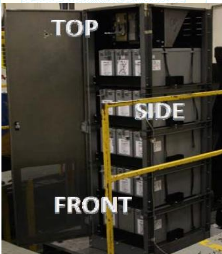
Overall view of UUT2
