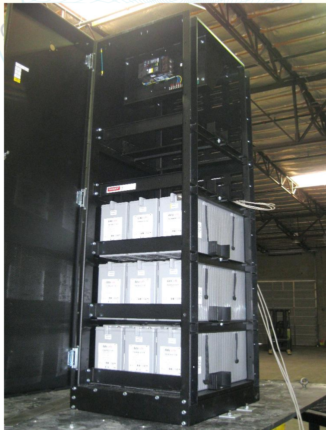
Overall view of UUT4
