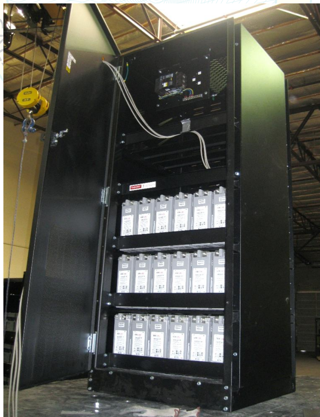
Overall view of UUT3
