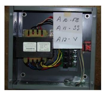
Rigid wall mounted to wall fixture with (4) 5/16" cap screws. Unit maintained structural integrity and remained functional per manufacturer requirement after shake table test. Contents were included in testing per operating conditions.
