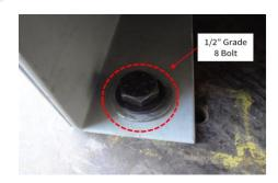
Base mounted-rigid using four (4) 1/2" -13 SAE Grade 8 bolts with lock washers and flat washers. Unit maintained structural integrity and remained functional per manufacturer requirement after shake table test. Contents were included in testing per operating conditions.
