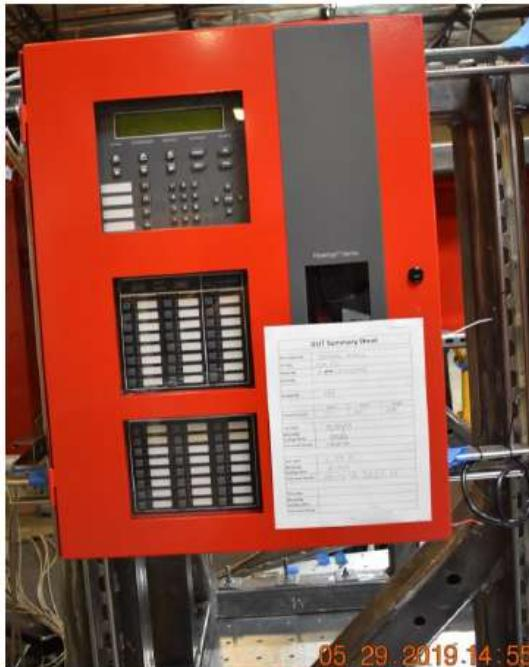
All units were filled with contents and maintained structural integrity and functionality after AC-156 test.
