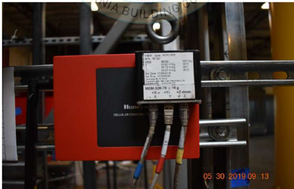
All units were filled with contents and maintained structural integrity and functionality after AC-156 test.
