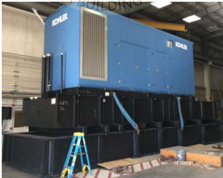
All units were filled with contents and maintained structural integrity and functionality after AC-156 test.
