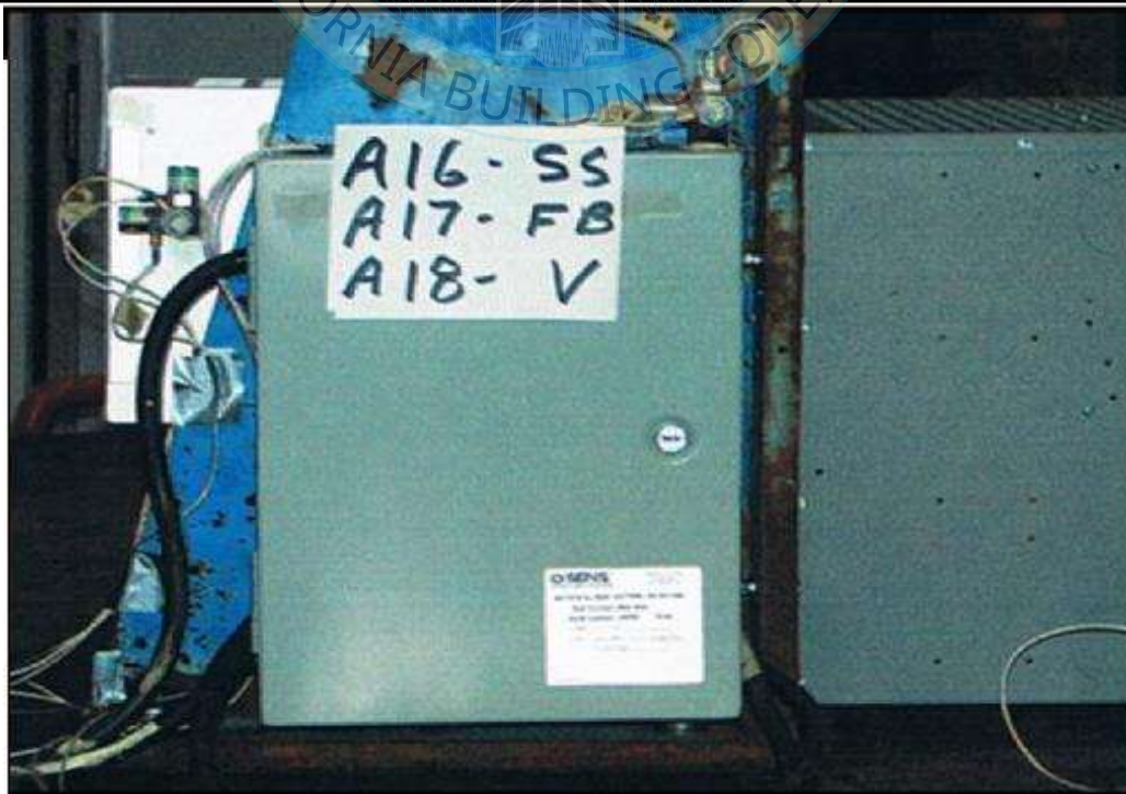
Overall view of UUT 6
