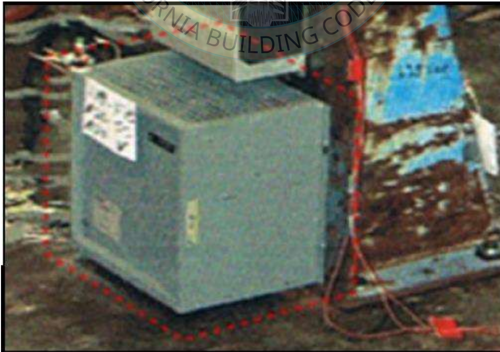
Overall view of UUT 3
