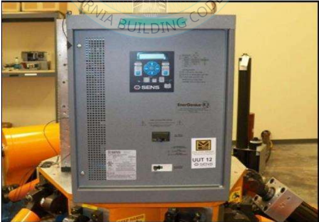
Overall view of UUT 12
