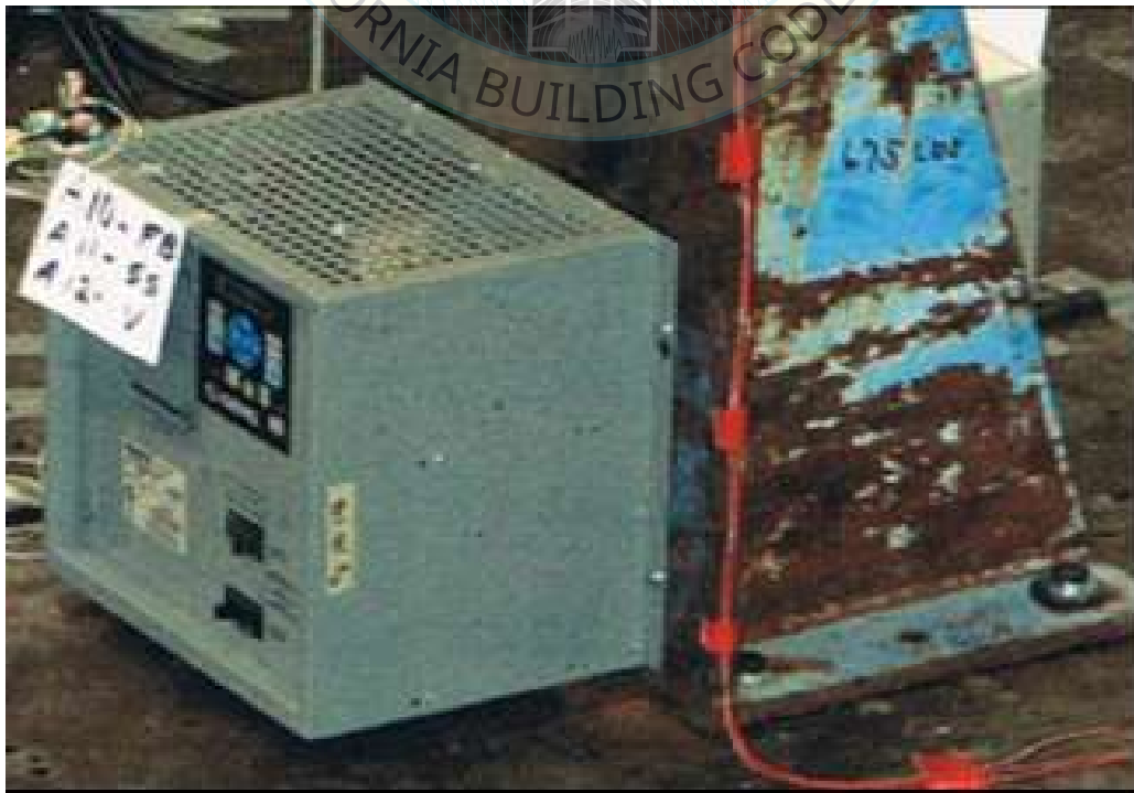
Overall view of UUT 4
