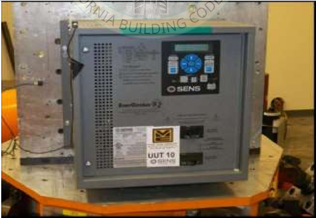
Overall view of UUT 10
