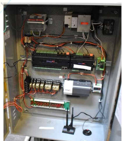
Interior view of panel
