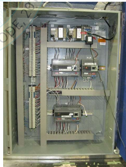
Interior view of panel
