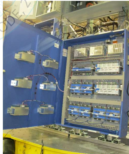
Interior view of panel
