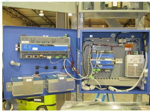
Interior view of panel
