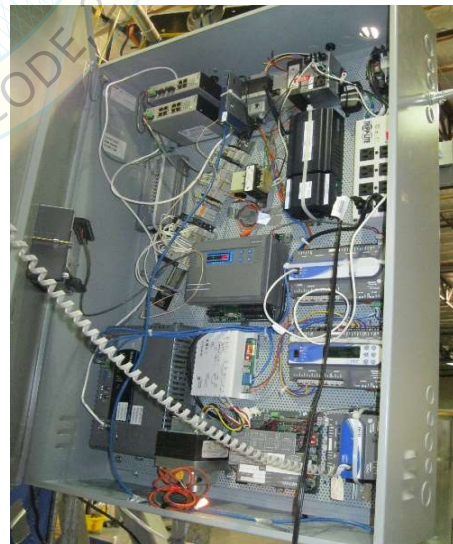
Interior view of panel
