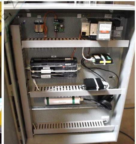
Interior view of panel
