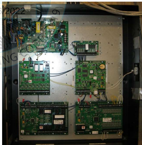
Interior view of panel
