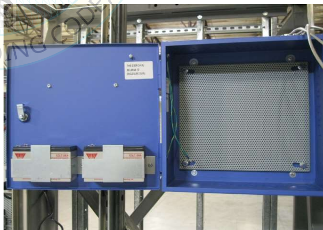
Interior view of panel
