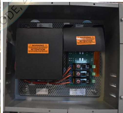
Interior view of panel
