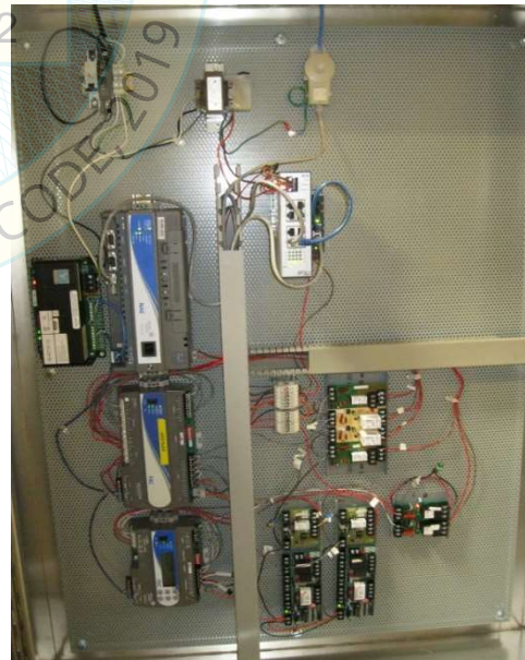
Interior view of panel
