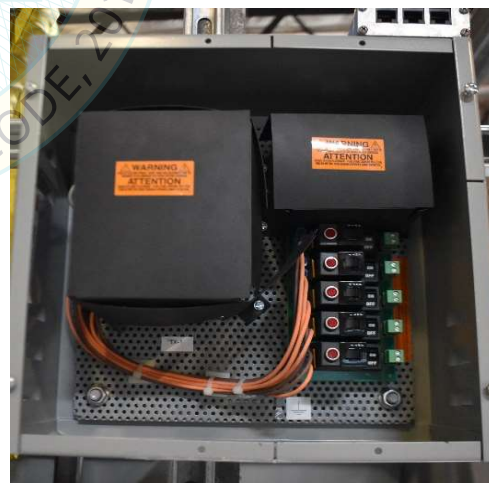
Interior view of panel
