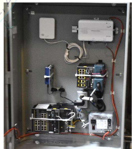
Interior view of panel
