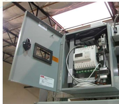
Interior view of panel
