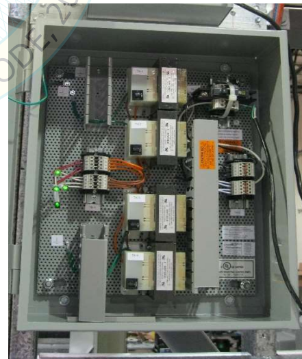
Interior view of panel
