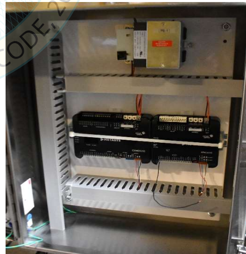
Interior view of panel
