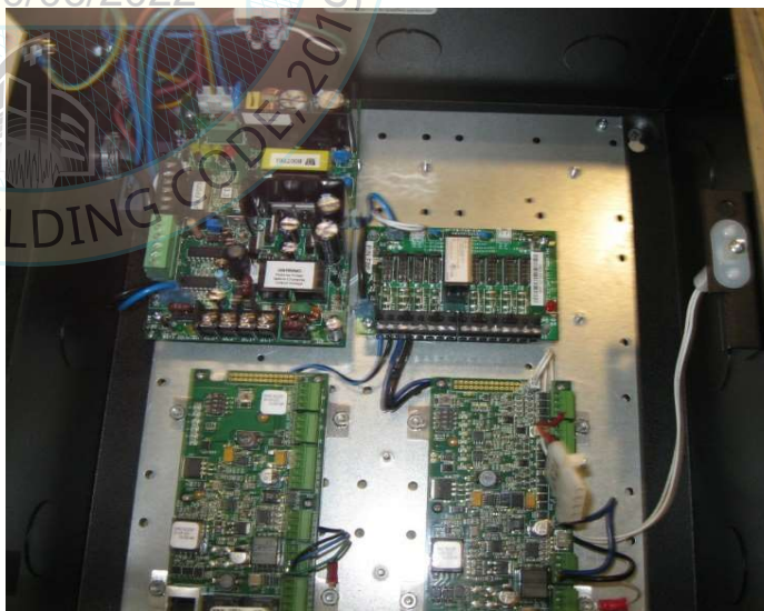
Interior view of panel
