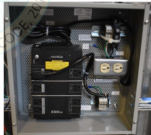
Interior view of panel
