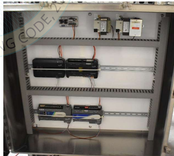
Interior view of panel
