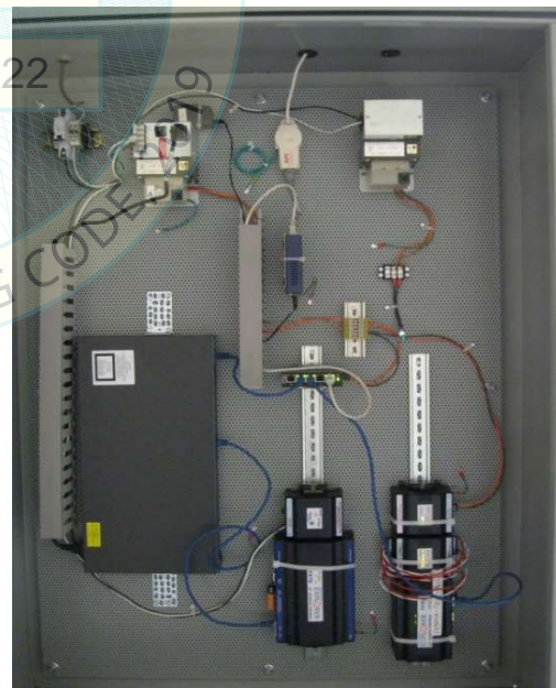
Interior view of panel
