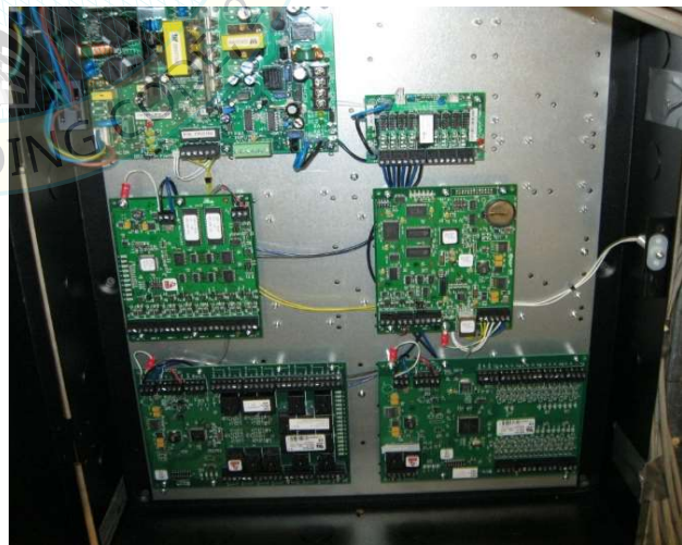
Interior view of panel
