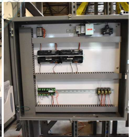
Interior view of panel
