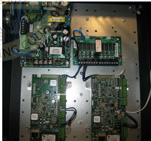
Interior view of panel
