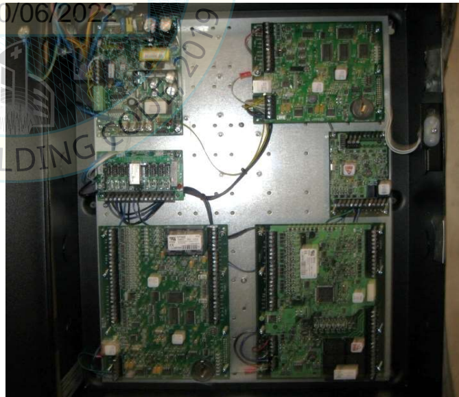
Interior view of panel
