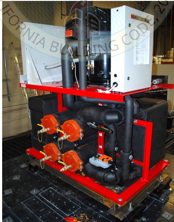
Overall view of UUT-09
