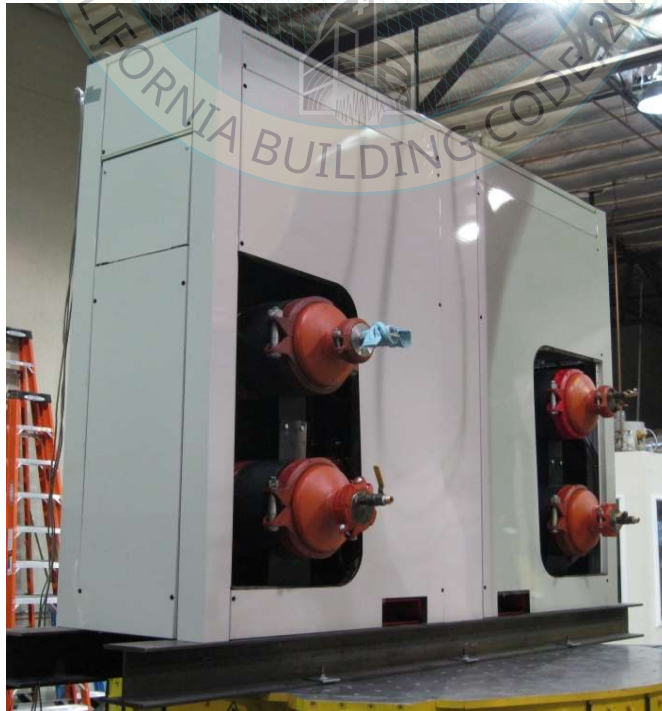
Overall view of UUT-07
