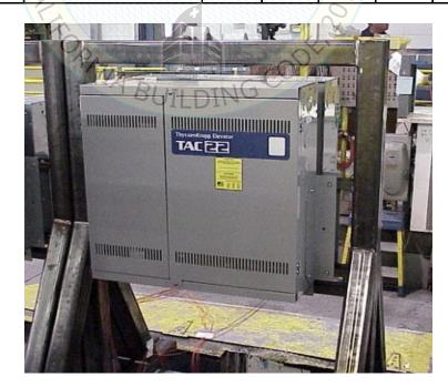
Wall Mounted - Rigid to fixture using six (6) 3/8"-16 Grade 5 bolts and washers.
