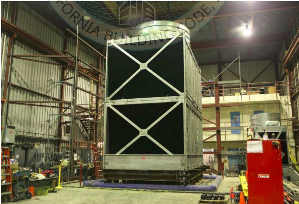
All units were filled with contents and maintained structural integrity and functionality after AC-156 test.
