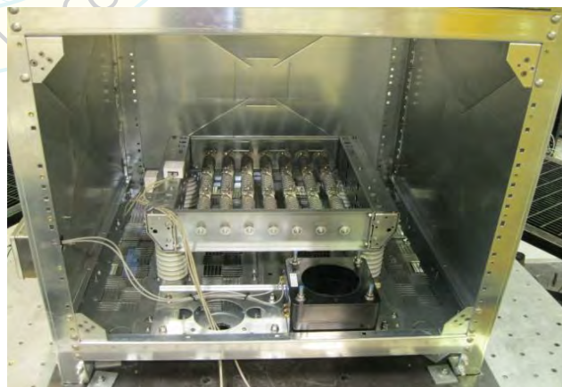
UUT-03B interior view.
