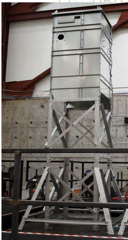
UUT-06B overall view.
