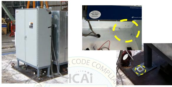
Attached to support platform using ten (10) 1/2 in. A307 bolts. Support platform bolted to ground using four (4) 1/2 in. A307 bolts (one per support leg) B-line FW-1/2" 17/32 thick, Carbon steel Electro Galvanized Flat Washer. Base Plate B200-Square Washer 1-5/8 Sq. by 1/4" Thick
