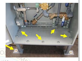
Attached to support platform using ten (10) 1/2 in. A307 bolts. Support platform bolted to ground using four (4) 1/2 in. A307 bolts (one per support leg) B-line FW-1/2" 17/32 thick, Carbon steel Electro Galvanized Flat Washer. Base Plate B200-Square Washer 1-5/8 Sq. by 1/4" Thick
