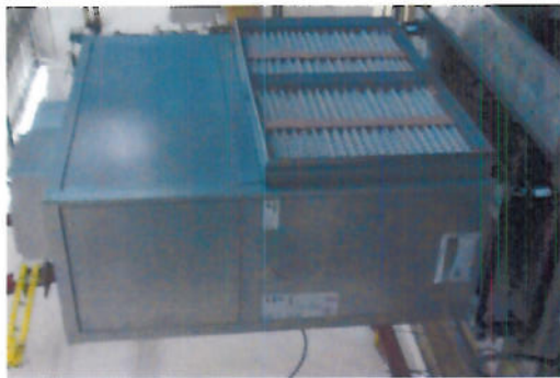
VBY40, Base Mounted on AMSR-1C Isolators
