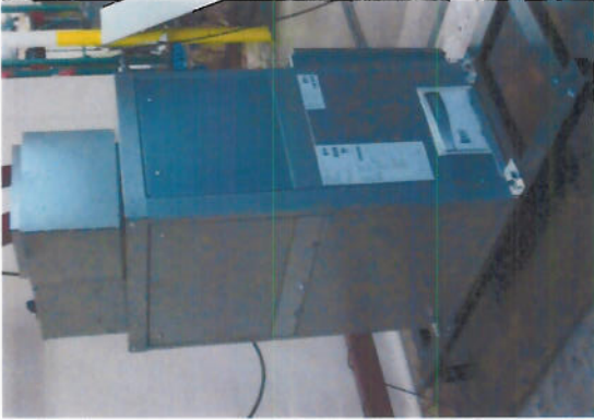
VBY06, Base Mounted on AMSR-1C Isolators
