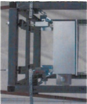
HLY20, suspended with HRS-1C hanger boxes
