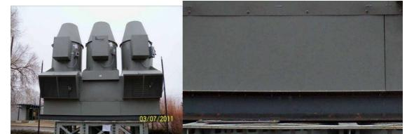
The unit was anchored using fasteners centered on the 5" curb flange with 7.5" center to center between screws. 5/16"-24 Dril-Flex Self Drilling/Tapping Screws with 3/16" Min. thread engagement into A36 steel with 5/8" min. edge distance were used.
