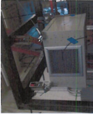
HLC06, suspended with HRS-1C hanger boxes
