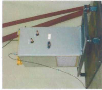
HLC06, suspended with HRS-1C hanger boxes
