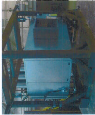
THB12, suspended with HRS-1C hanger boxes
