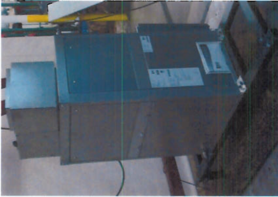
CW06, Base Mounted on AMSR-1C Isolators
