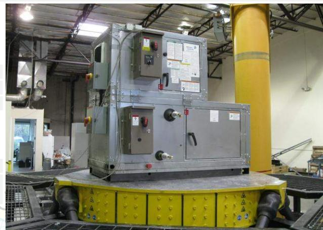
Mounting: Base mounted rigid using #14 sheet metal screws spaced at 7.5-in o.c. around the perimeter.
