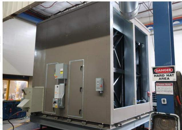
Mounting: Base mounted rigid using (12) 3/4-in diameter Grade 8 bolts. Each side wall (parallel to airflow) has (6) 6-in long L3x3x3/8-in brackets spaced 24-in o.c. Each bracket connects to the unit base with (2) 3/4-in diameter Grade 5 bolts.
