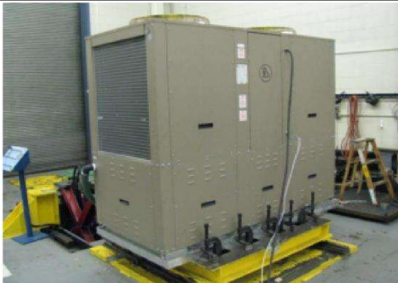
Overall view of UUT-03
