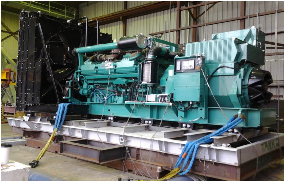
Equipment layout on table. Genset secured to a sub-base tank via (14) VMC M2SSH-1E-6500N spring isolators.
