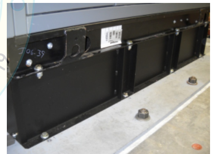
Figure 1B.2: Mounting Detail
