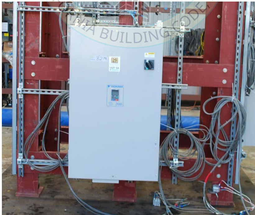
All units were filled with contents and maintained structural integrity and functionality
