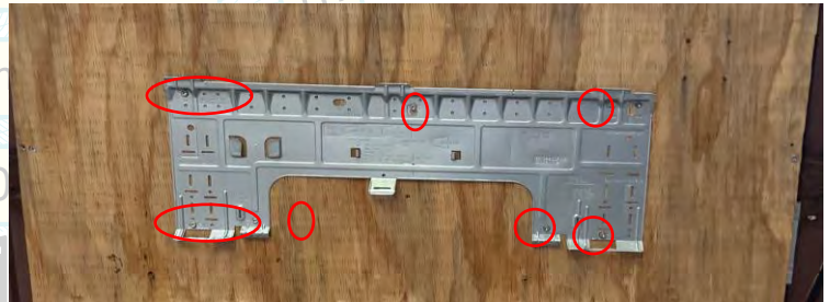
UUT73 wall plate to wall fastener locations
