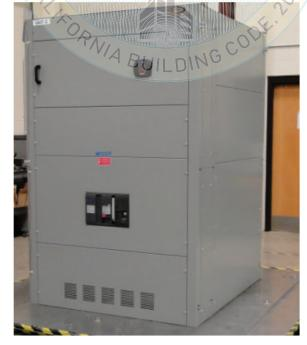
UUT 2 was rigid base mounted with (6) 1/2" grade 5 bolts. The bolts are spaced approximately 53" lengthwise and 22.5" widthwise on center.
