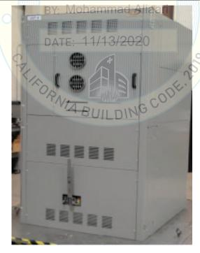
UUT 4 was rigid base mounted with (6) 1/2" grade 5 bolts. The bolts are spaced approximately 53" lengthwise and approximately 22.5" widthwise on center.
