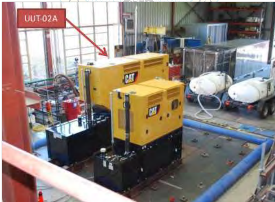
Unit tested with empty tank and maintained structural integrity and functionality after AC-156 test.
