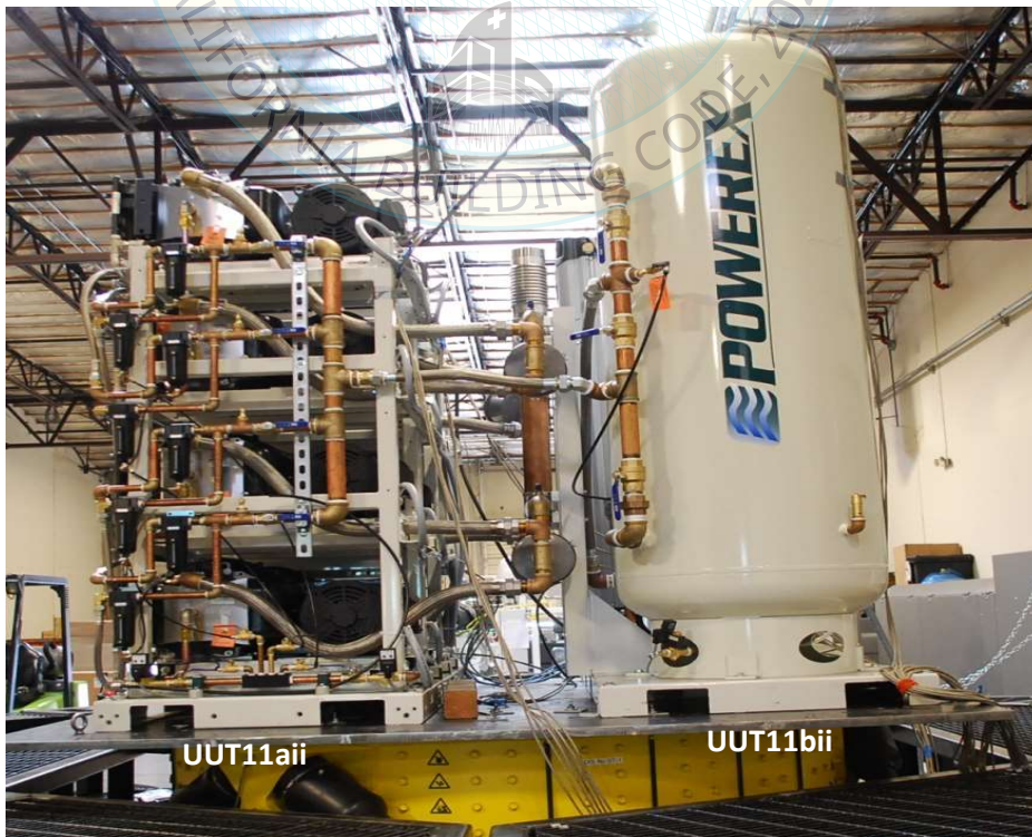
UUT11aii, UUT11bii Overall View
