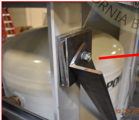
Brace attachment detail
