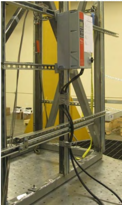
Overall view of UUT1a
