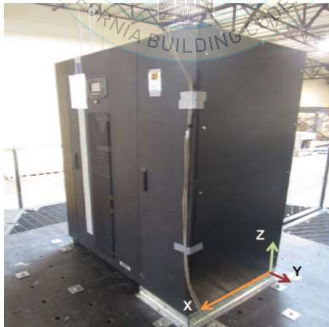
All units were filled with contents and maintained structural integrity and functionality after AC-156 test.
