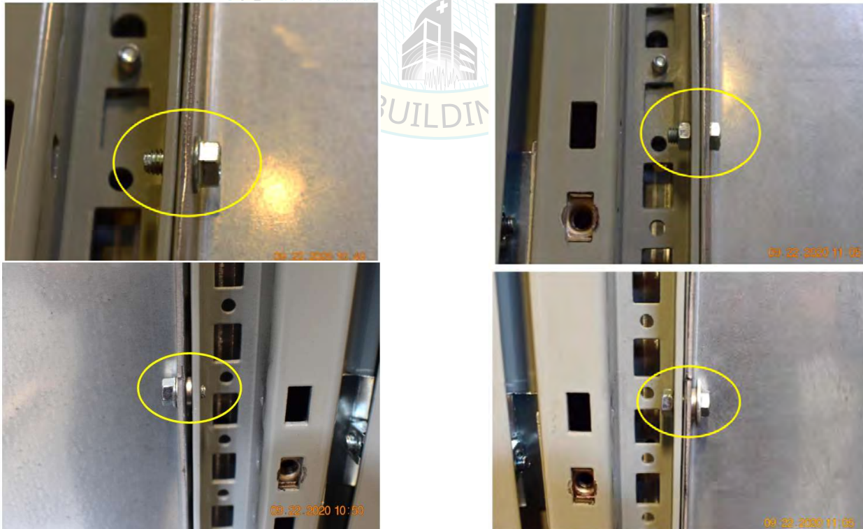
All units were filled with contents and maintained structural integrity and functionality after AC-156 test.
