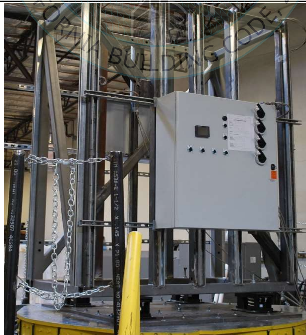
UUT18B Overall View
