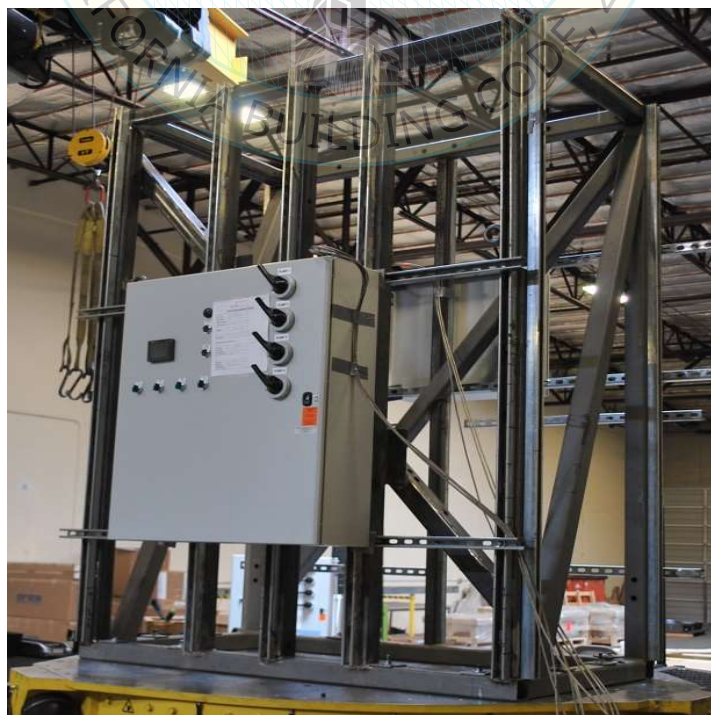
UUT18A Overall View
