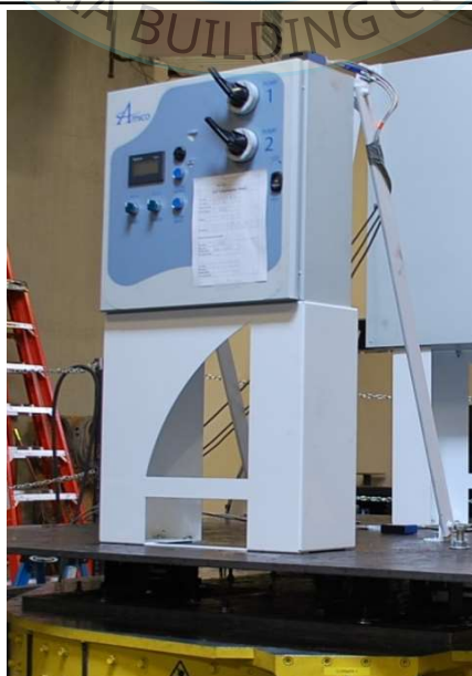
UUT19B Overall View
