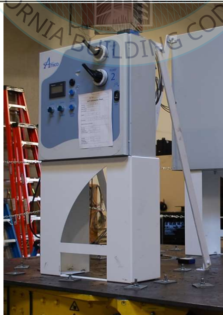
UUT19A Overall View
