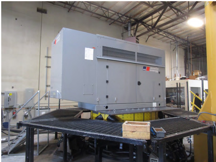
All units were filled with contents and maintained structural integrity and functionality
