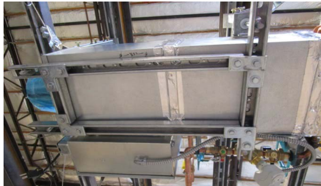
View of bottom strut support
