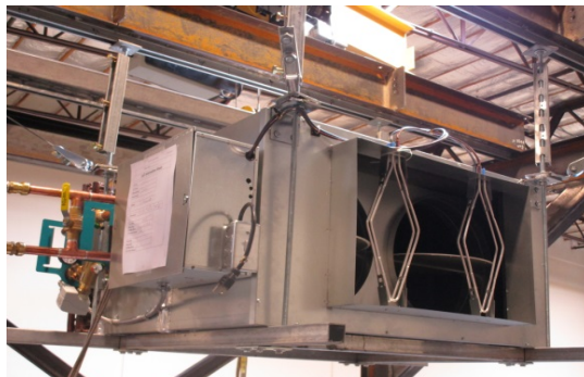
Overall view of unit
