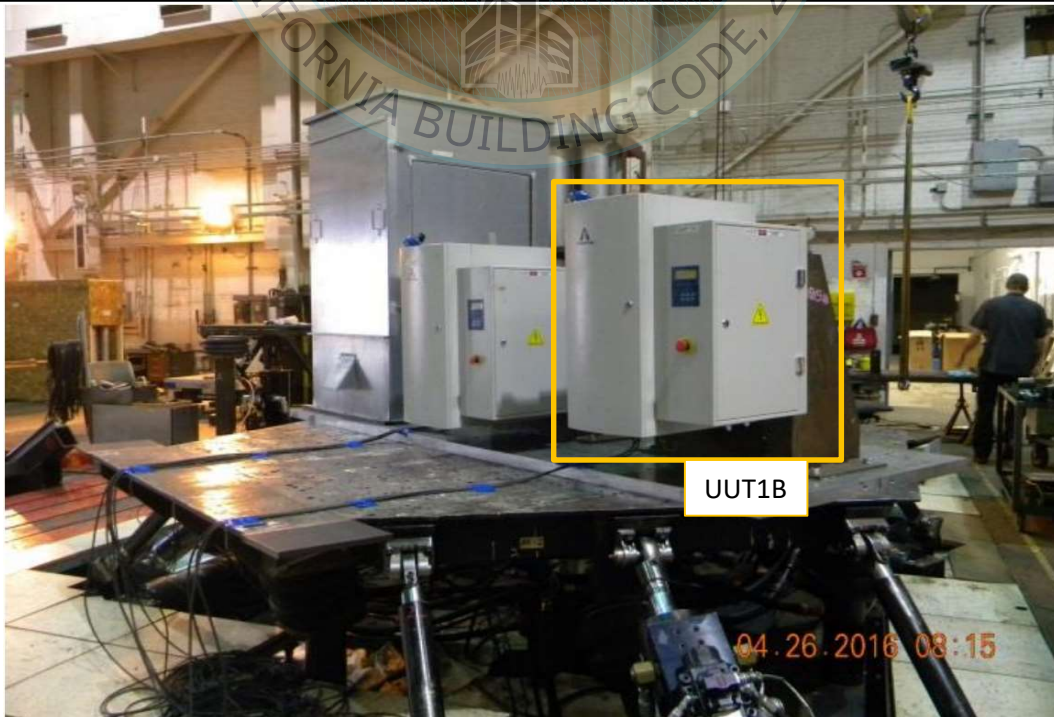
Overall view of UUT1B.2 (Wet)
