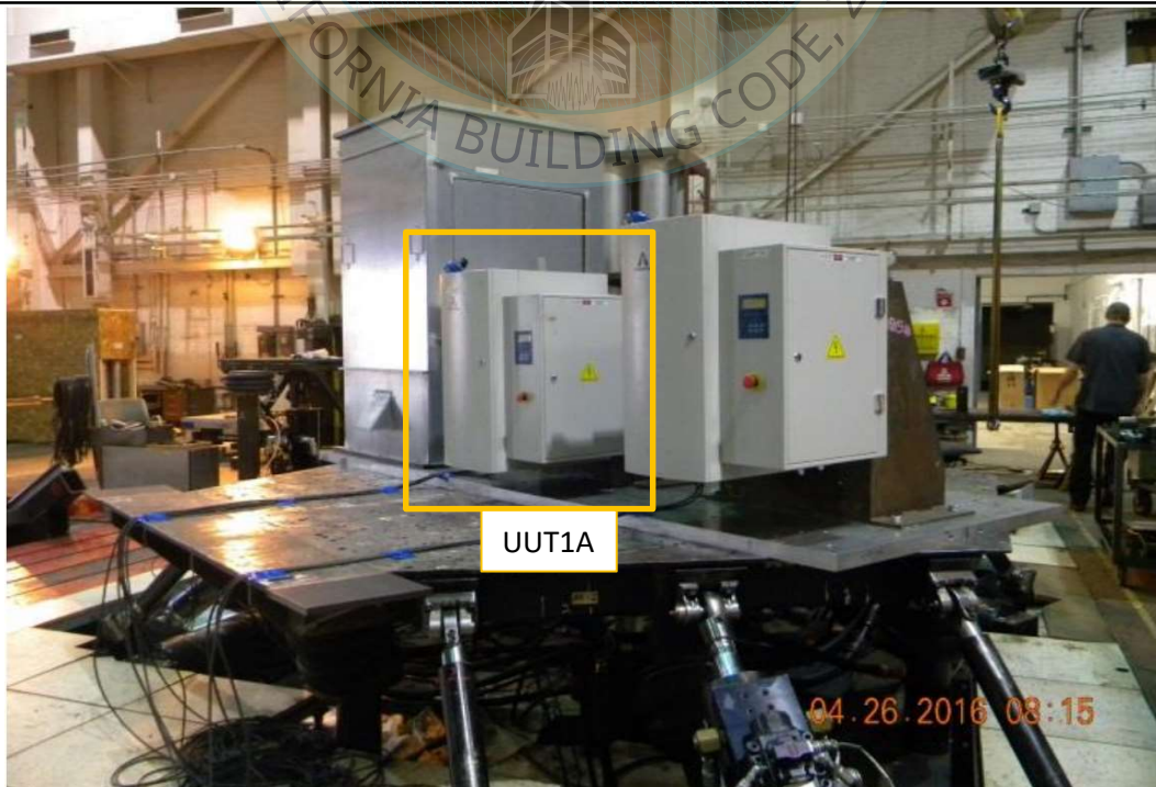
Overall view of UUT1A.2 (Wet)
