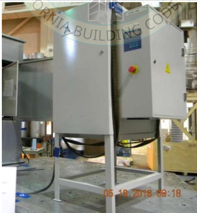
Overall view of UUT3B.2 (Wet)
