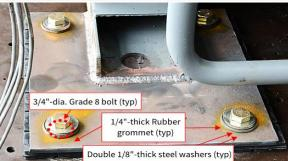
Base mounted on (4) 12x16x3/8" A36 steel plates with 22" of 3/16" fillet weld each. Base plates and channel are fully supported by Vibrex ISOCUBE 3/4" thick neoprene pads. Base plates are anchored using (4) 3/4" Grade 8 bolts each.
