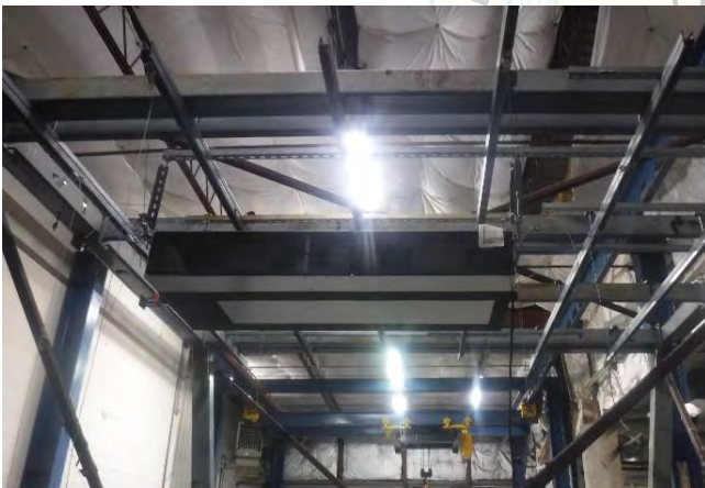
Two Mason SCB/SCBH-0 Braces per hanging rod.
