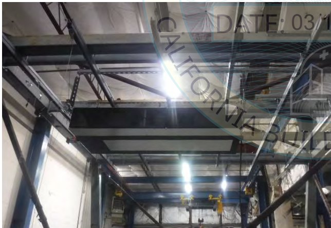
Two Mason SCB/SCBH-0 Braces per hanging rod.
