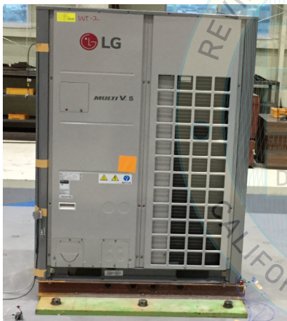
Figure UUT-A2.1: Unit on the shake table
