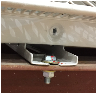
Figure UUT-D4.3: Anomaly - screw fell
