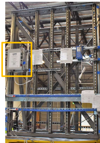
Figure 1. Overall view of UUT-08a
