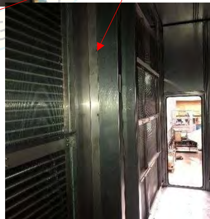
#12-3/4" self tapping screws @ 12" OC along length of blankoff and (5) self tapping screws in base and ceiling panel (typical)
