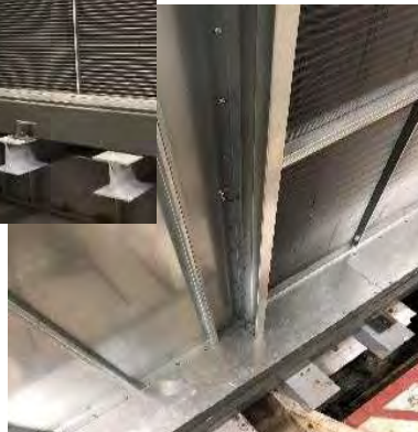
#12-3/4" self tapping screws @ 12" OC along length of blankoff and (5) self tapping screws in base and ceiling panel (typical)
