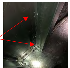
#12-3/4" self tapping screws @ 12" OC along length of blankoff and (5) self tapping screws in base and ceiling panel (typical)
